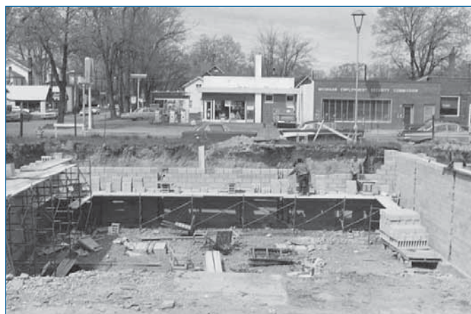
Construction of 31 South Howell Street Office Circa 1968
