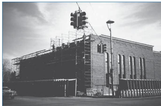
Construction of One South Howell Street Office 1987
