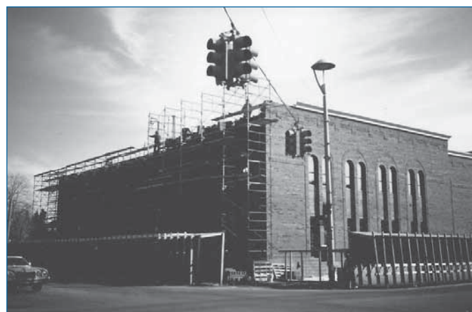
Construction of One South Howell Street Office 1987
