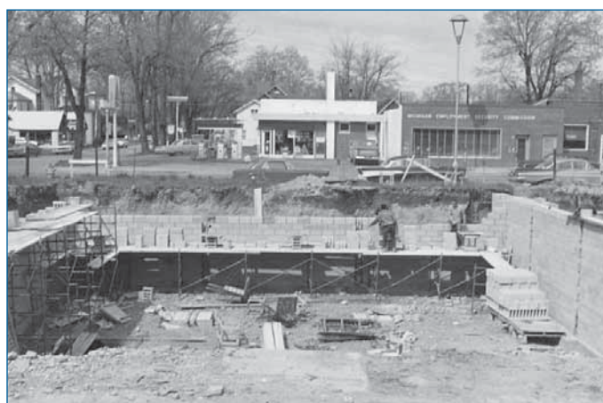
Construction of 31 South Howell Street Office Circa 1968
